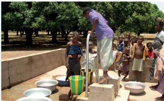
Footpump in rural Burkina Faso
