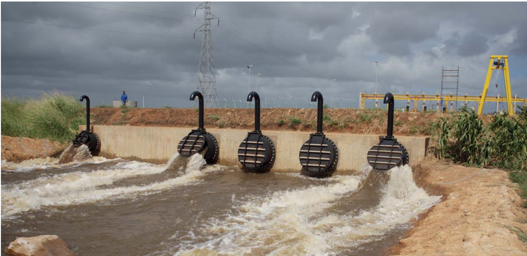
Flap valves of the Massingir dam, Mozambique
