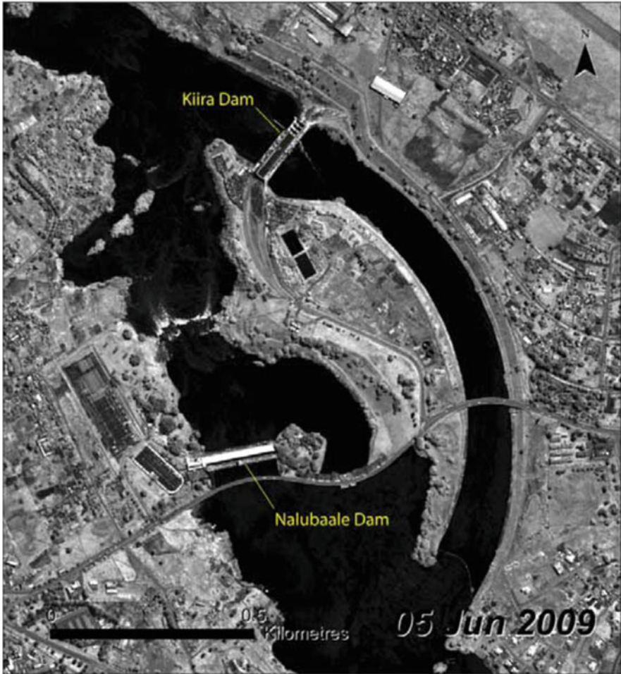
Fig. 14 Nalubaale and Kiira dams in Uganda (Google Earth 2009)
